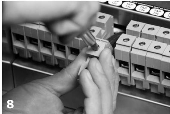
8 Insert wire(s) into terminal back and tighten.
