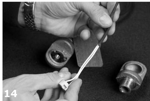
14 Remove old socket from insulation sleeve.
