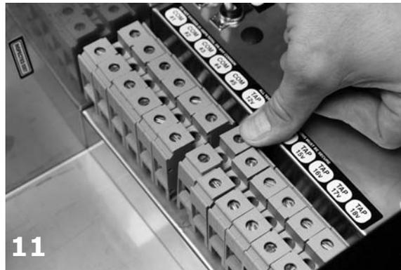
11 Apply pressure to front and back to secure.
