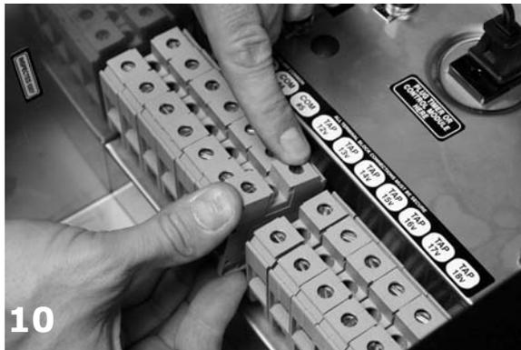
10 Press terminal block into place - back first.
