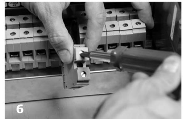
Unscrew tap screw to remove terminal.
