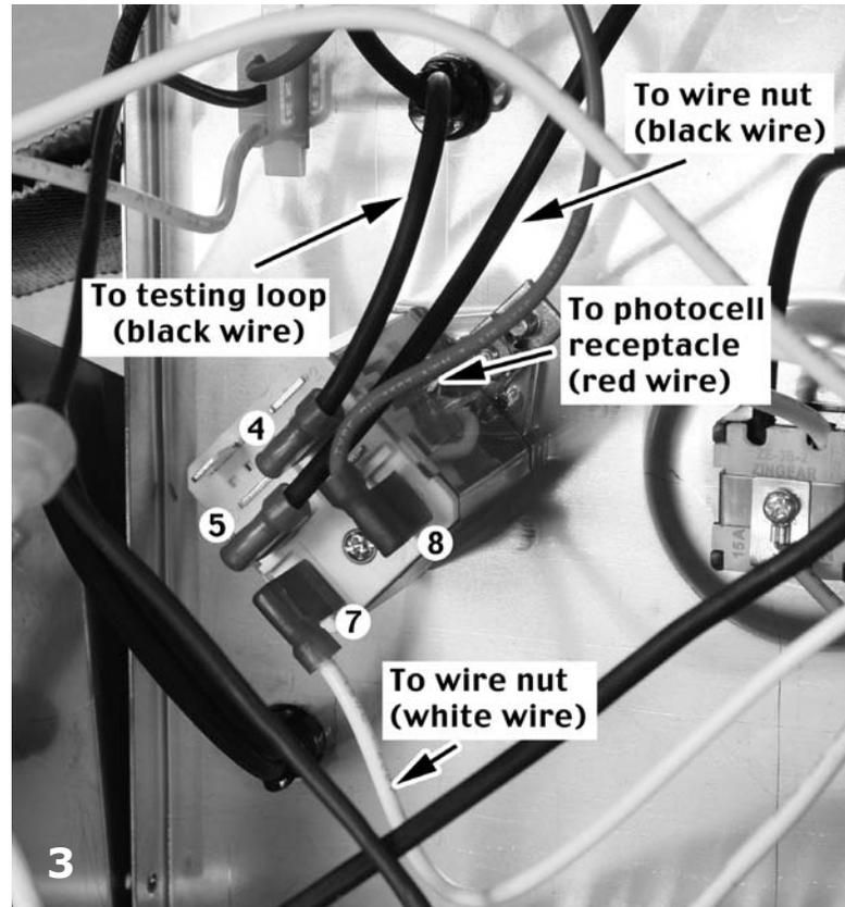
3. Locate the Power Bypass Relay (see picture 3).
