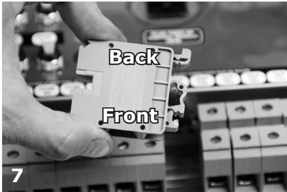
7 Replace terminal noting correct direction.
