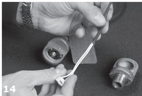
14 Remove old socket from insulation sleeve.
